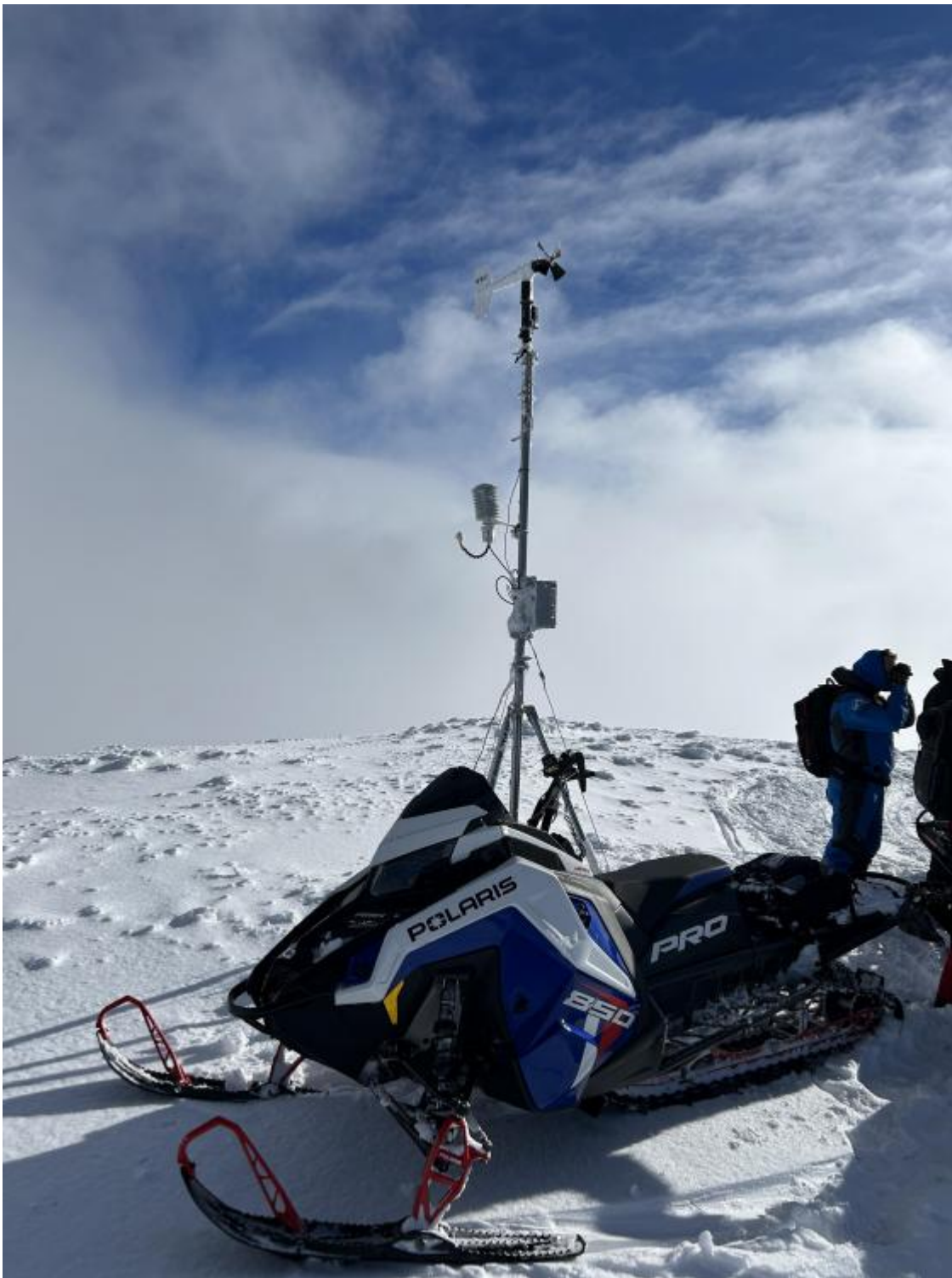
De-iced Sawtell anemometer
